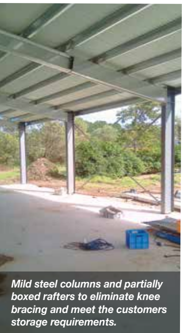
7.5m wide bays achieved with cold-form steel to provide optimum space for storing cotton bales in between portal frames.
